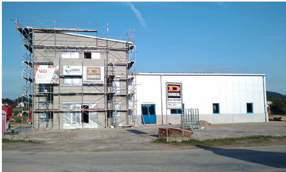
Construction area in Cham, Germany, opening spring 2011
